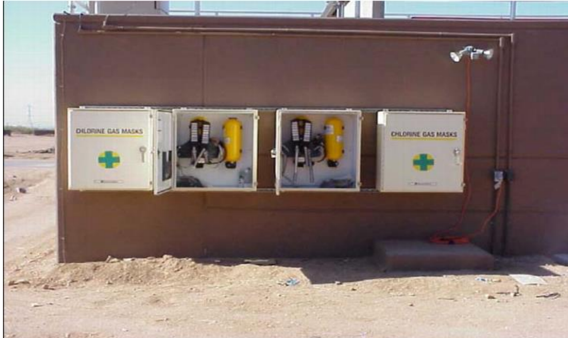
Figure 22: Respirators Shall Be Available Outside the Chlorine Building
